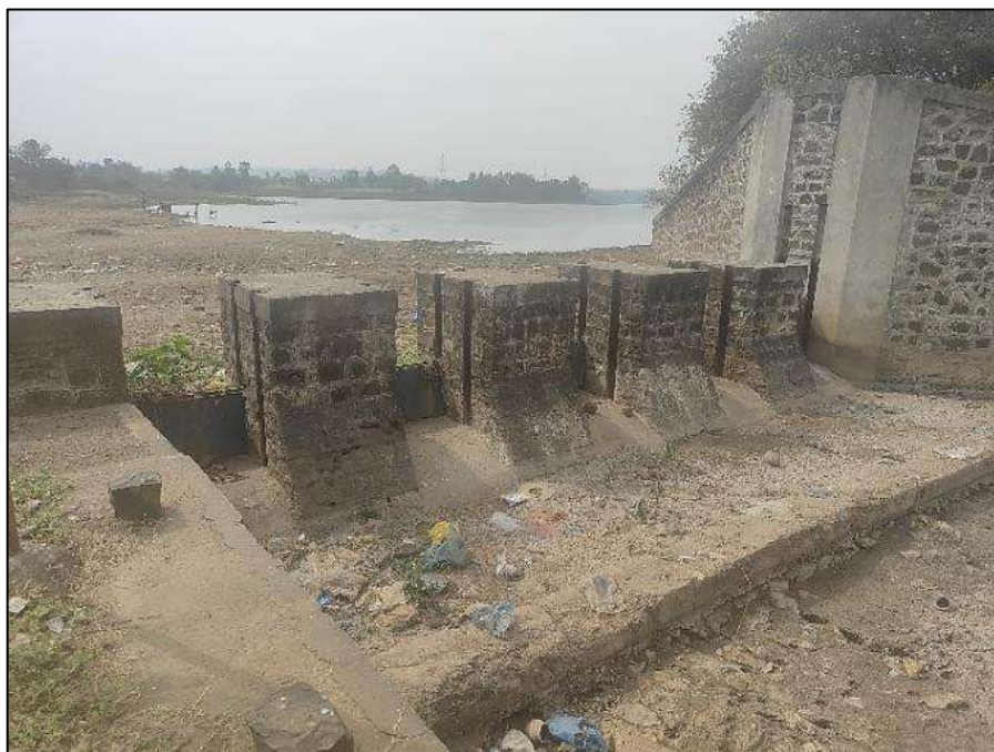
Figure 2-11: Kalamba Lake Proposed Sluice Gate
